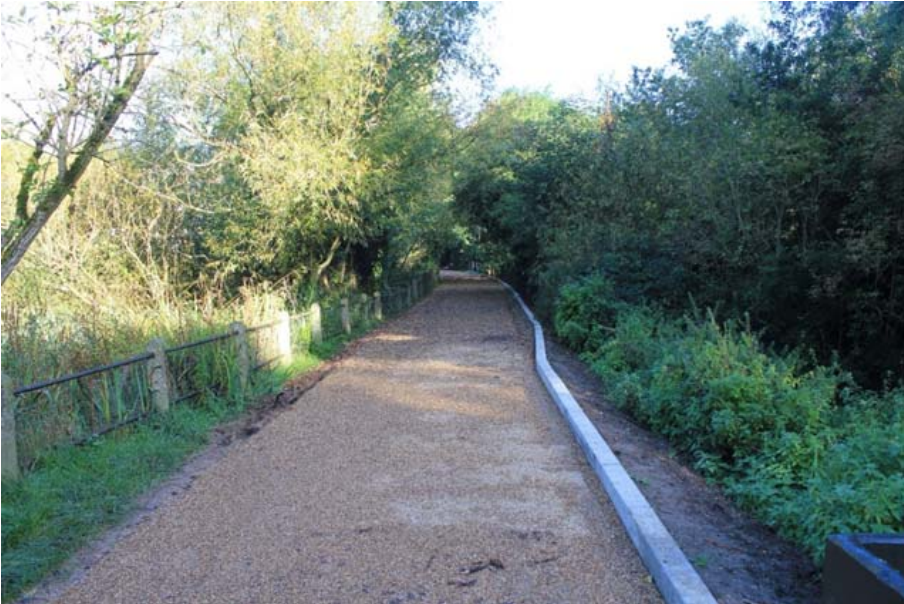
Picture 5 - Completed works at Vale of Health
