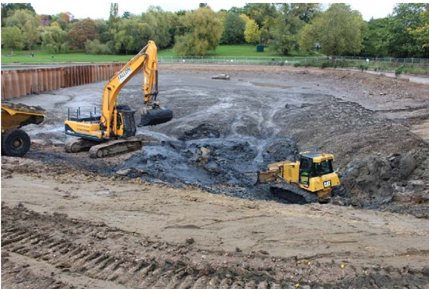
Picture 2 - De-silting Model Boating Pond using excavators
